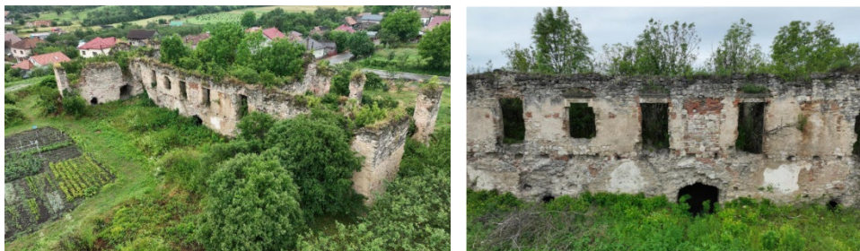
Fig. 4. Current condition of the ruins of Bocskai Castle in Aghireșu. Left: aerial view of the ensemble; right: view of the surviving walls.
