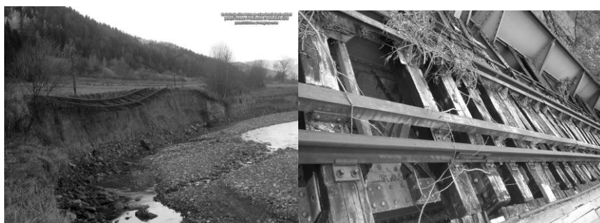
Fig. 3. The Rădăuți - Brodina railway after the 2008 floods (photo: Porcuțan, A.)
