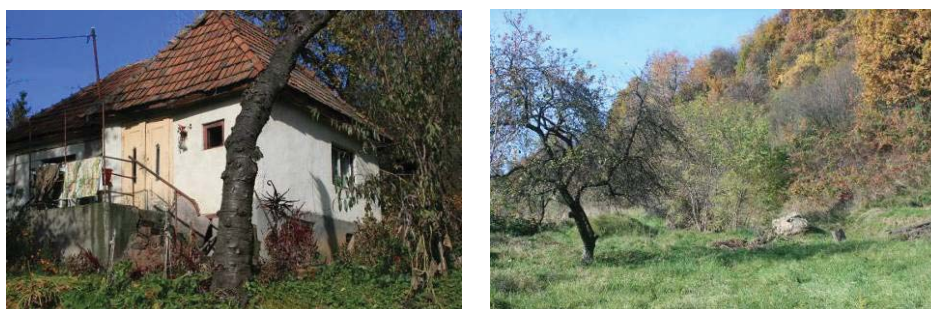
Figure 5. Landslide from Plaiului street
