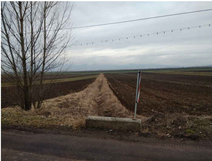
Fig. 3. Agricultural constructions for the prevention of rainfall on the slopes and the protection of the road near Fișag stream.
