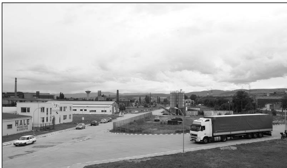
Foto 4. Industrial Park Hunedoara (Source: replicahd.ro )
