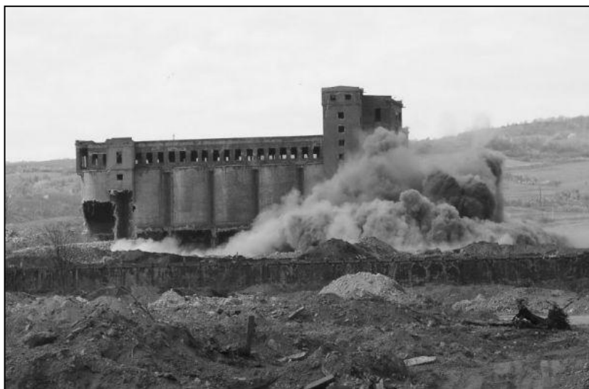
Foto 5. Demolition on the steel platform ( Source: evz.ro )
