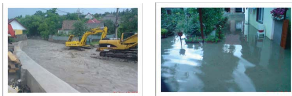
Figure. 2. Valea Racilor Brook overflows, together with pluvial flooding in June 2010
