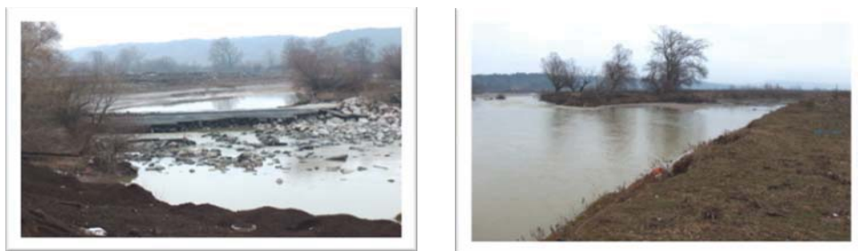
Figure.1. Arieș River diversion for the December 2009 flooding and damage to water mains from Mechel enterprise.
